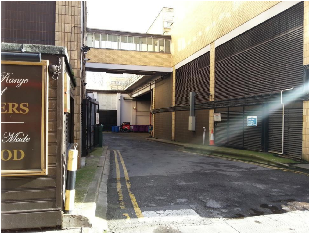
Photo 1 - View from Porchester Road – 13 February 2013
