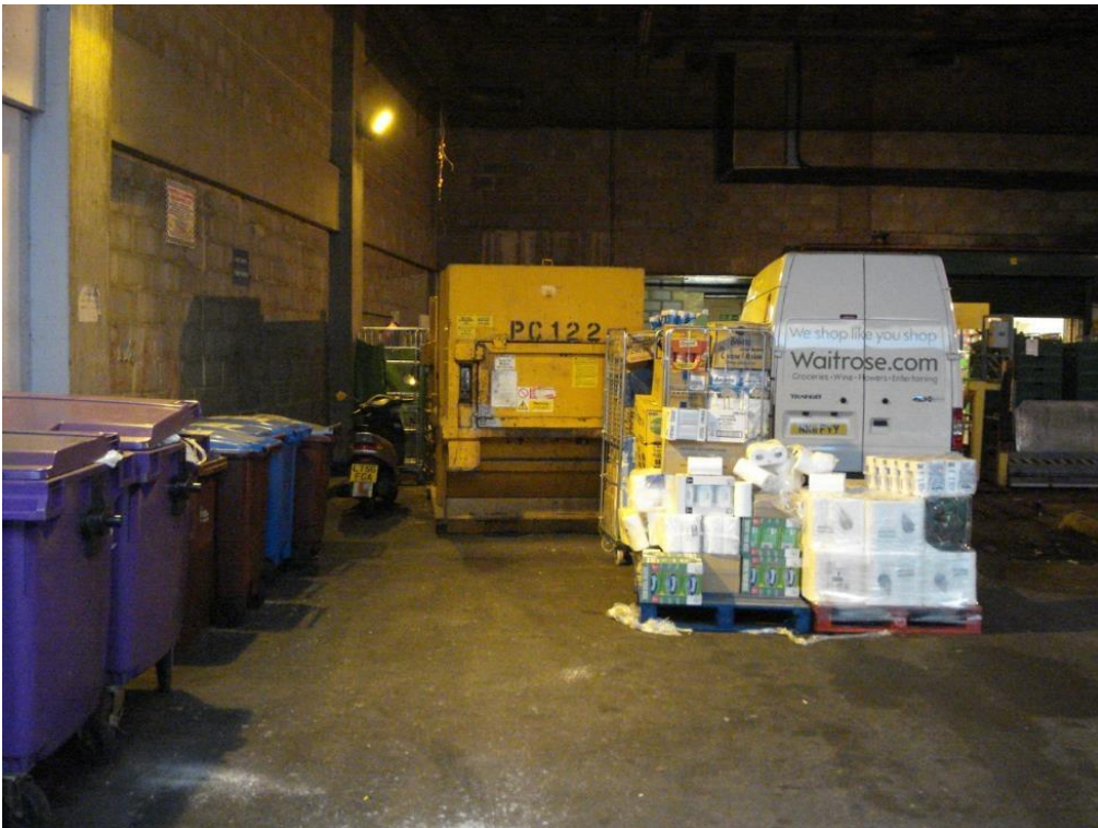
Photo 3 – View into Covered Service Yard (2 of 3) – 17 February 2013
